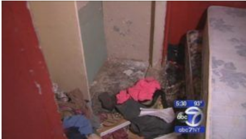
Deplorable conditions inside the Garden Spires complex. Photo courtesy of ABC
