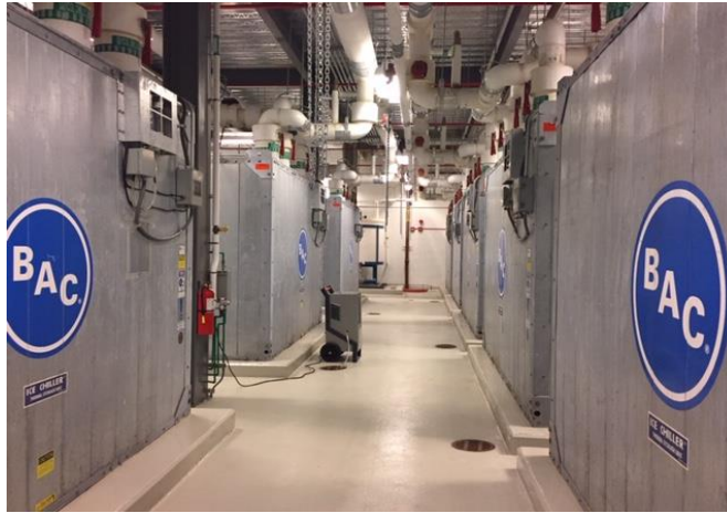
The frozen-water tanks to support A.C. to work more effectively.
