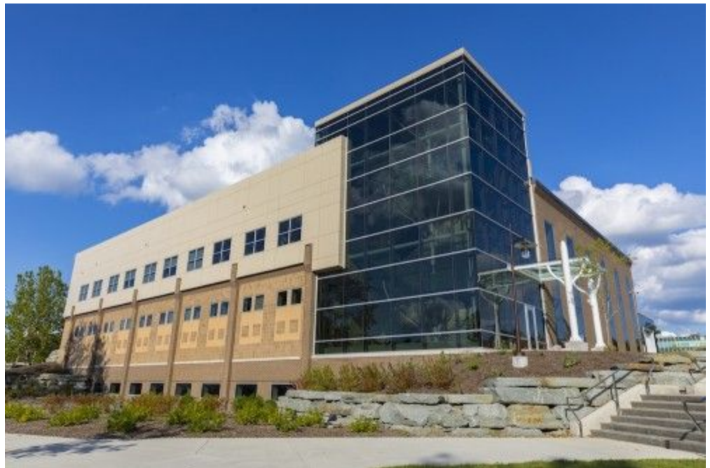
Smart Energy Research and Development Facility at Binghamton University
